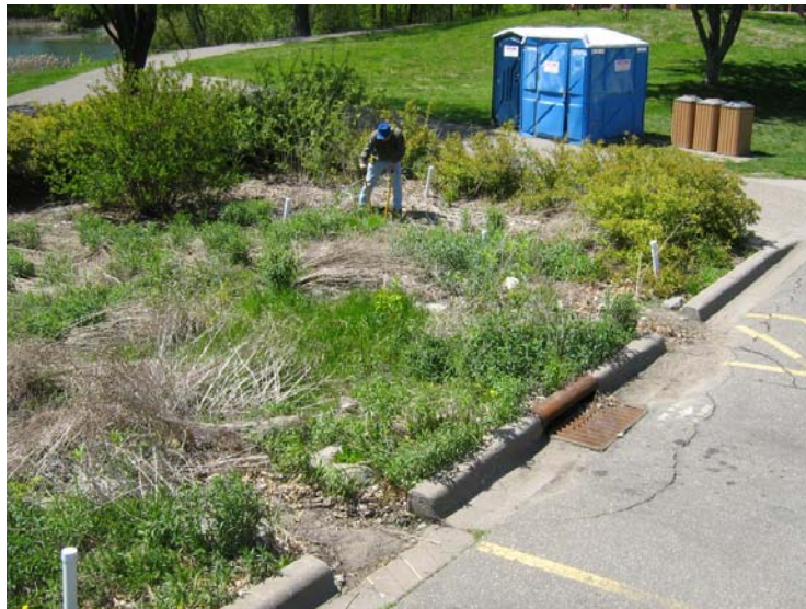
Figure 2-3. Photo of the Thompson Lake bioretention cell and curb-cuts during the growing season looking northwest.
