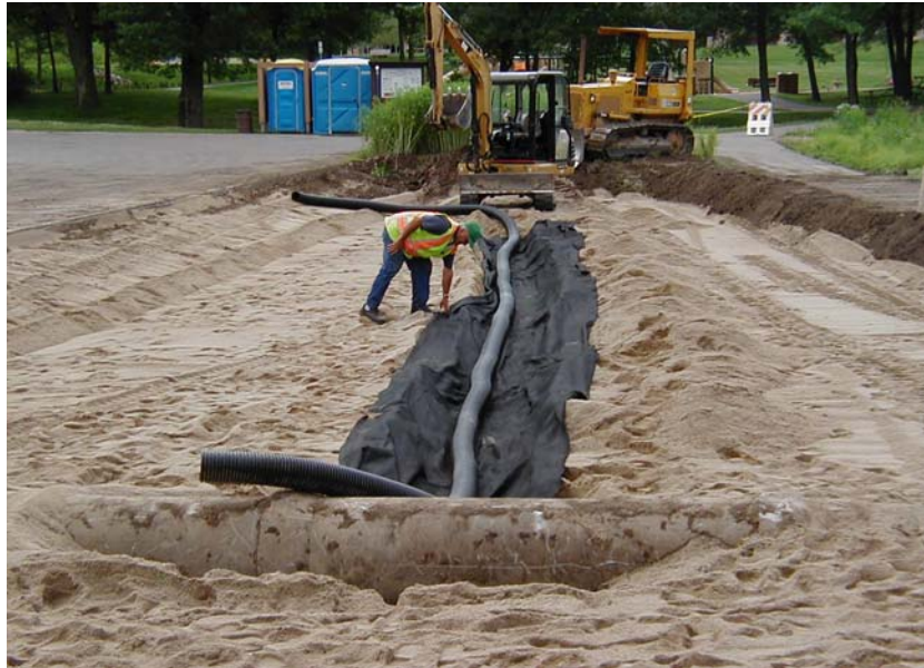
Figure 2-6. Photo (looking south) of the construction of the Thompson Lake bioretention cell under-drain installation above clay soils within the amended soil layer and connected to existing storm sewer.
