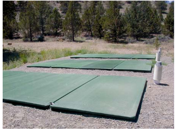
7,500 gpd AdvanTex recirculating packed media filter system. The AdvanTex system is similar to RSF/RGF's, but occupies a smaller footprint. Treatment media is housed in non-corrosive enclosed "pods". The modular design enables adding capacity over time for phasing-in developments and tracking flows. Courtesy of Orenco Systems, Inc.
