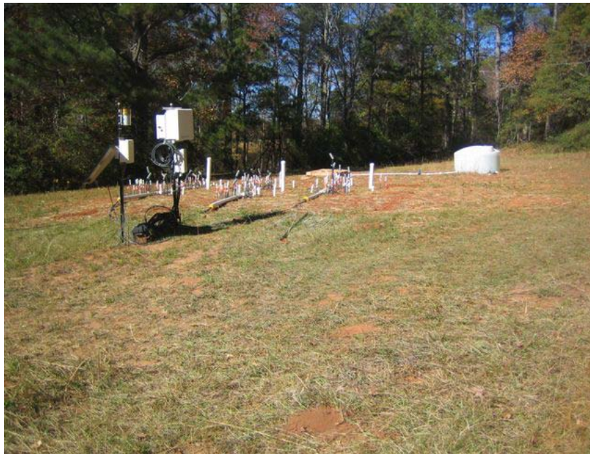
Figure C-1. Experimental UGA Site Showing Storage Tank that Discharges to the Septic Tank and Three Trenches and Instrumentation. A Data Logger Housing, Rain Gauge, and Solar Panel is Also Shown.
