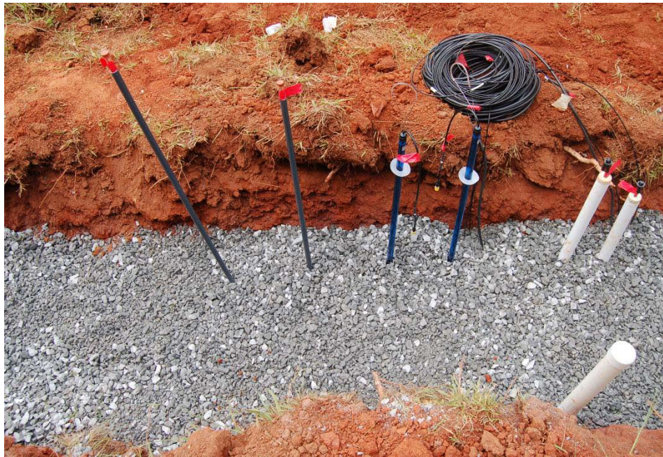
Figure C- 3. Trench During Installation of Sensors into the Underlying Soil.
