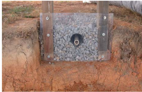
Cross section of an LPD trench (demonstration)
