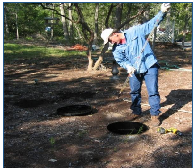
Service providers regularly measure depth of sludge and scum to determine when tanks need pumping.
