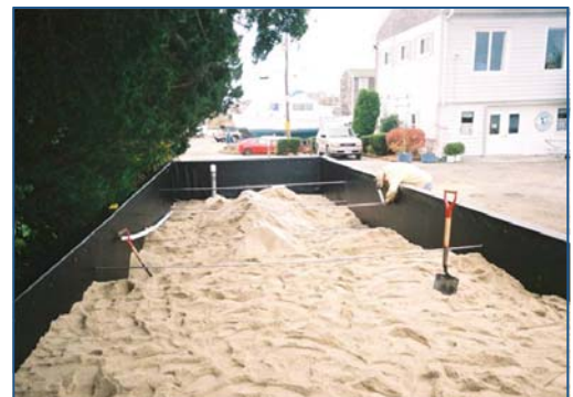
Sand or sand/gravel filters are generally constructed on the site
