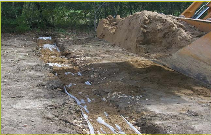
Trench installation showing geotextile fabric over washed rock media
