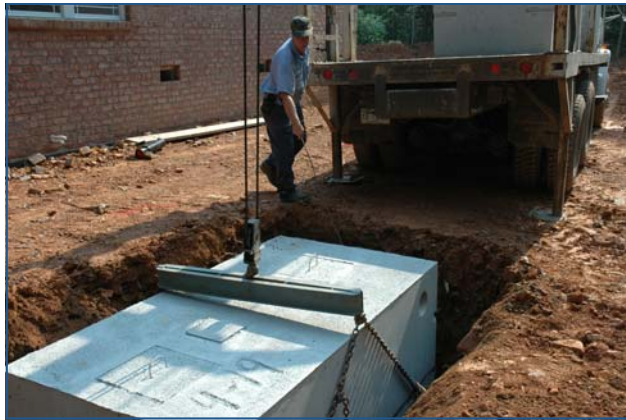
Installation of tanks requires reasonable site access for heavy equipment.
