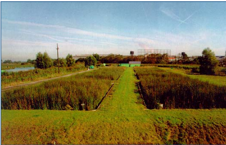
Parallel cells offer the flexibility to vary flow and loading.
