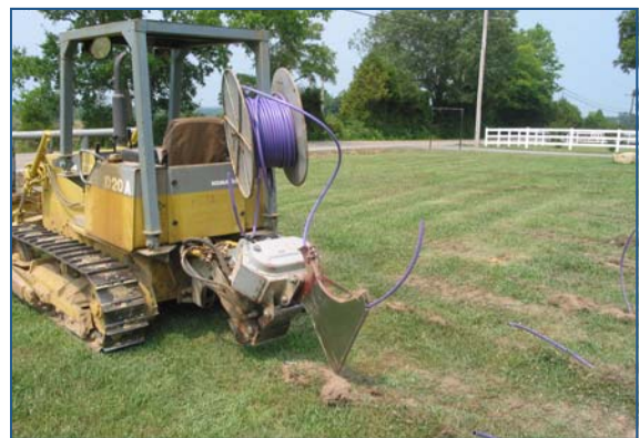
Installation of drip tubing using a vibratory plow
