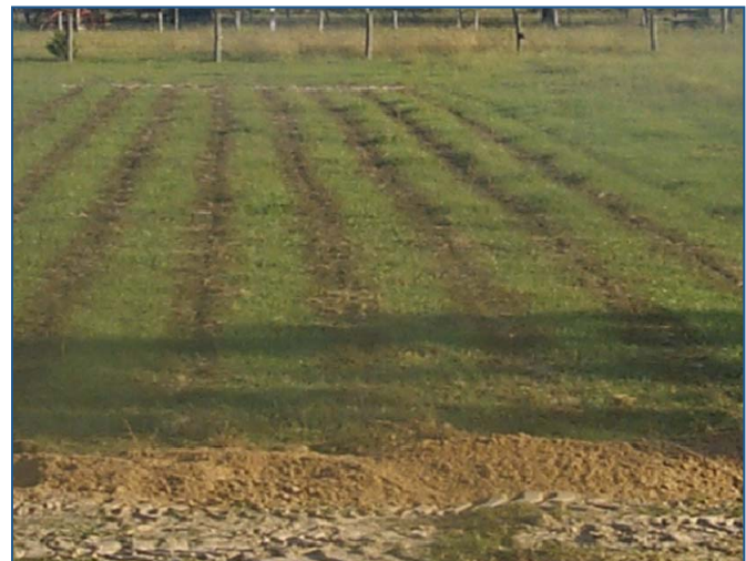
Installation of drip tubing itself results in minimal site disturbance. However, additional disturbance will result from installation of associated components such as septic and dosing tanks.
