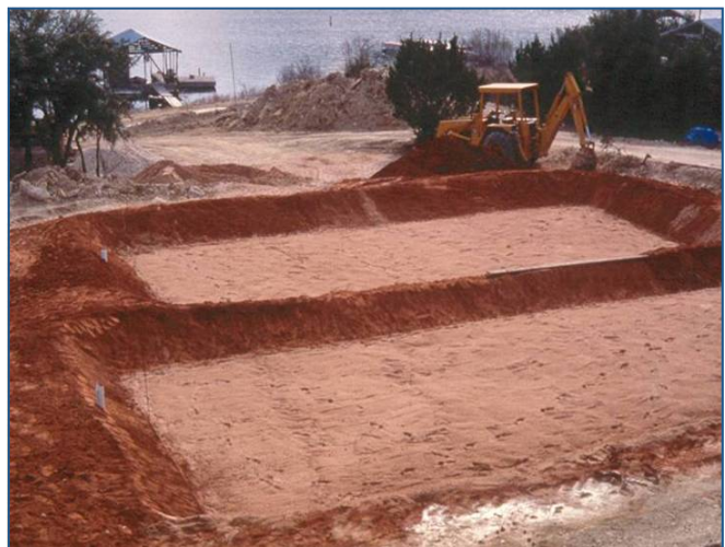
ET beds and ponds are constructed by making a shallow excavation and installing a plastic liner (above). If soils are clayey, the plastic liner may be omitted (below).
