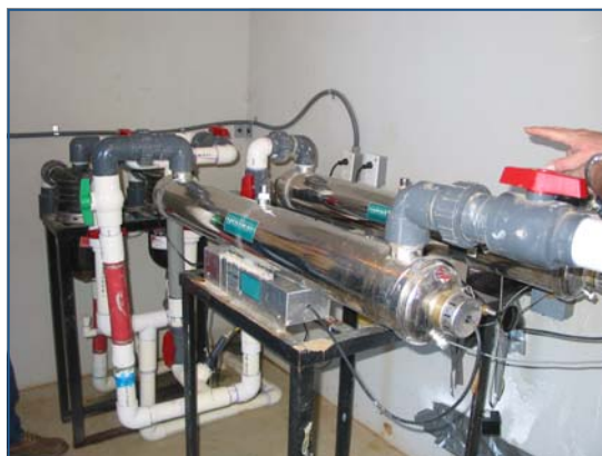
O&M for wastewater reuse systems depends upon the system components and the intended use. Unrestricted reuse will require a disinfection method such as chlorination (above) or Ultraviolet light (below). As with all components, regular O&M by qualified professionals is required.
