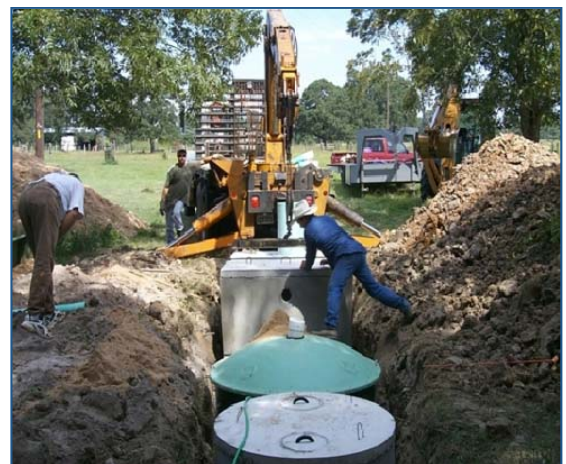
Alternately, components for suspended growth treatment can be installed inside tanks like those shown below.
