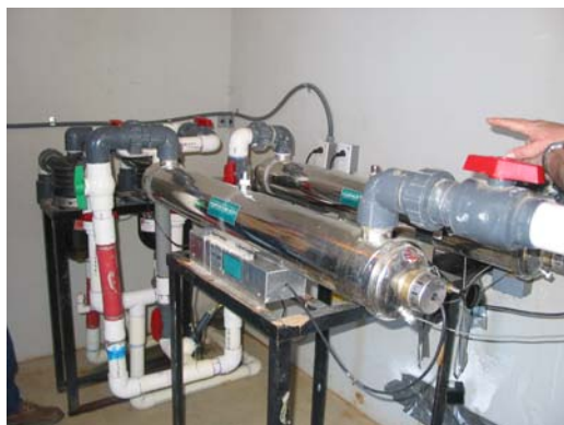
UV light is generated by passing an electrical charge through mercury vapor. This unit has a horizontally-oriented bulb.
