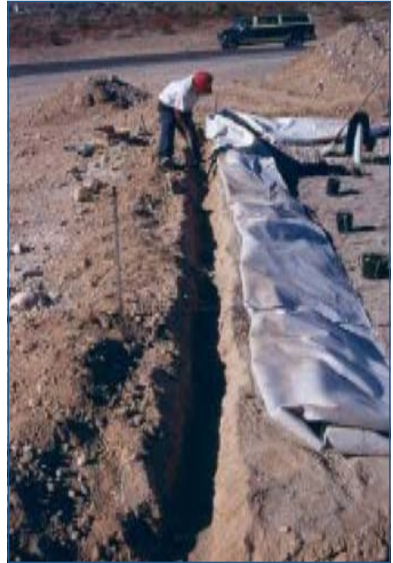
Installation of HDPE liner during construction of a wetland cell
