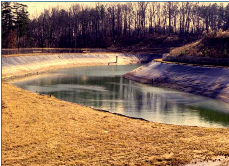
Lagoons can treat flows as large as a million gallons per day.
