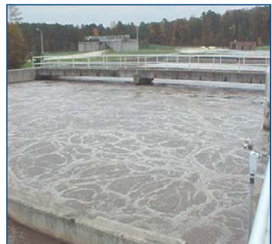
Residuals accumulate in septic tanks (above) and are also generated through suspended growth treatment processes like activated sludge (below).
