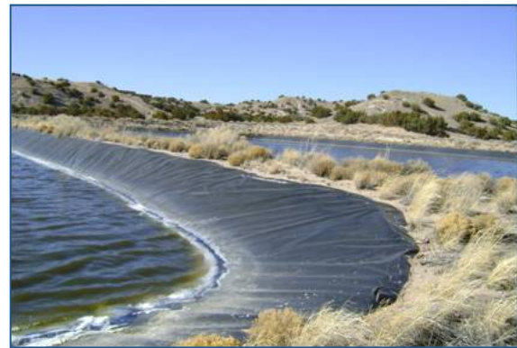
Evapotranspiration (ET) pond with a plastic liner
