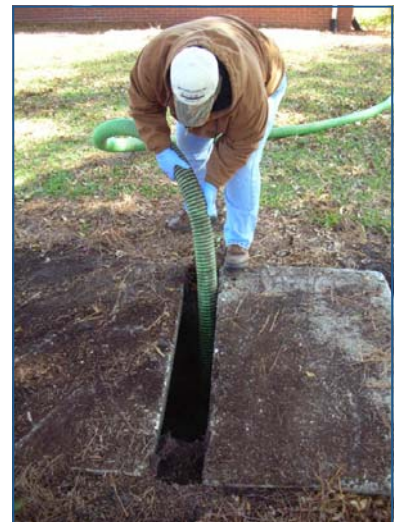
Residuals accumulate in septic tanks (above) and are also generated through suspended growth treatment processes like activated sludge (below).
