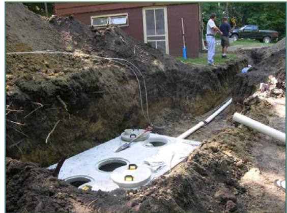
Installation of tanks requires reasonable site access for heavy equipment.
