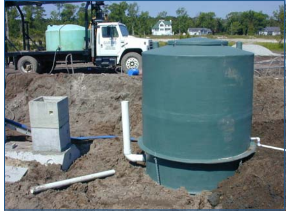
Suspended growth systems may be modular such as the units shown above and below.
