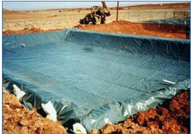
ET beds and ponds are constructed by making a shallow excavation and installing a plastic liner (above). If soils are clayey, the plastic liner may be omitted (below).
