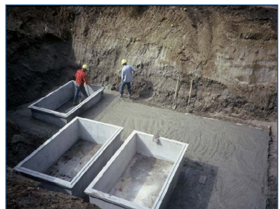
Alternately, components for suspended growth treatment can be installed inside tanks like those shown below.
