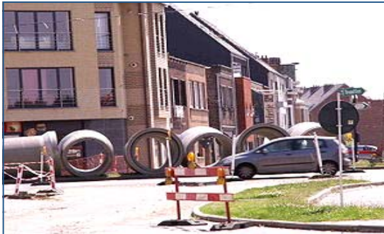
Gravity sewers require large diameter pipe.
