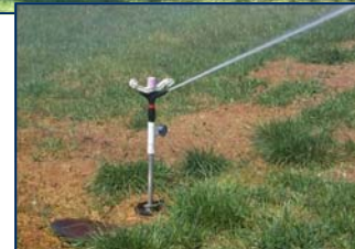
Residential spray irrigation system (above) and close-up of spray head (right)
