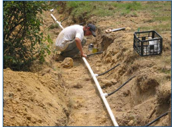
Once the drip tubing is installed, it is connected to a manifold.
