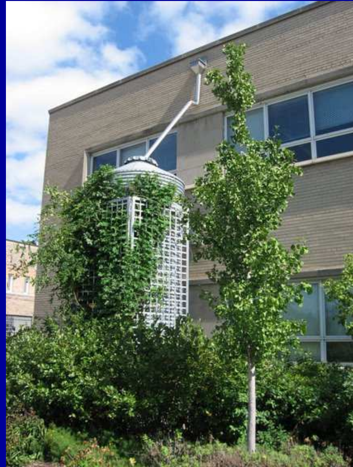
Cisterns collect rooftop runoff for reuse in Chicago. Credit: Abby Hall, USEPA
