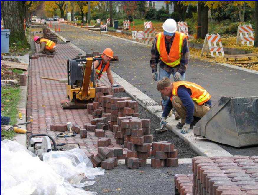
Installation of Permeable Pavers. City of Portland, BES
