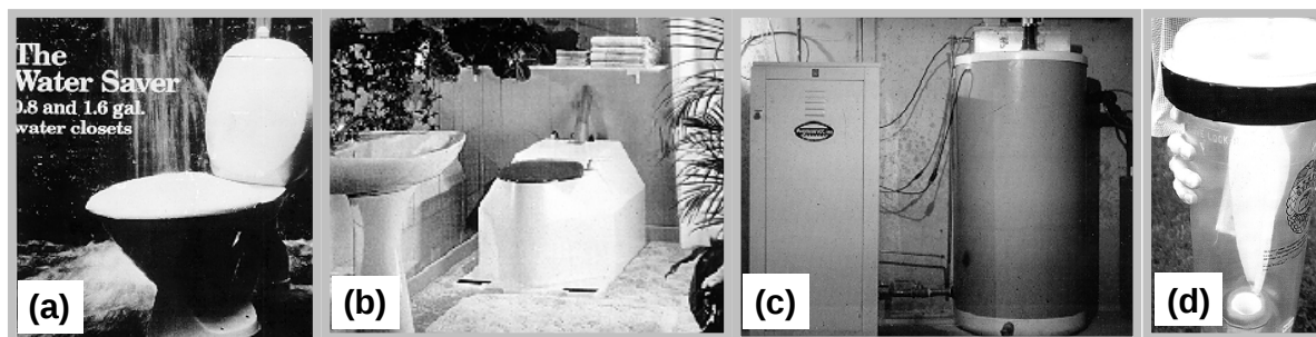
Fig. 6. Examples of wastewater source modifications: (a) 3-L volume flush toilet, (b) compost toilet, (c) graywater recycle unit, and (d) point-of-use bag filter for laundry discharge.
