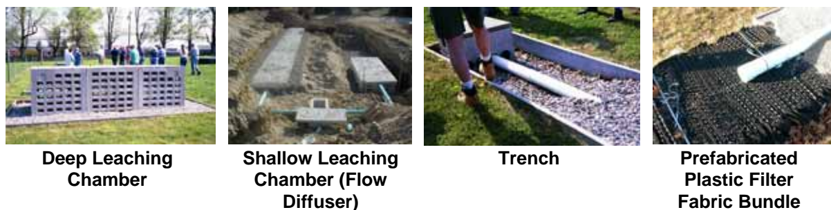
Figure 2-3 Typical Drainfield
