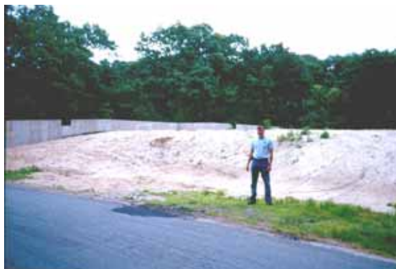
Figure 2-8 An Example of a Mound System That Is Five- to Six-Foot High
