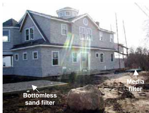
Figure 1-7 An Example of an Advanced Treatment System That Eliminates the Need for a Raised Leachfield
