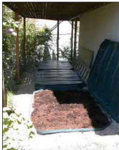
Figure 4-19 Modular Single-Pass Media Filters
