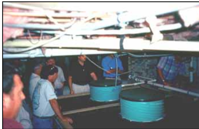
Figure 3-60 Septic Tank and Recirculating Media Located in the Building's Basement
