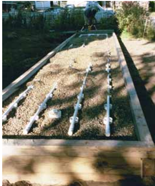
Figure 2-23 Bottomless Sand Filter Following a Recirculating Media Filter (multifamily/commercial use)
