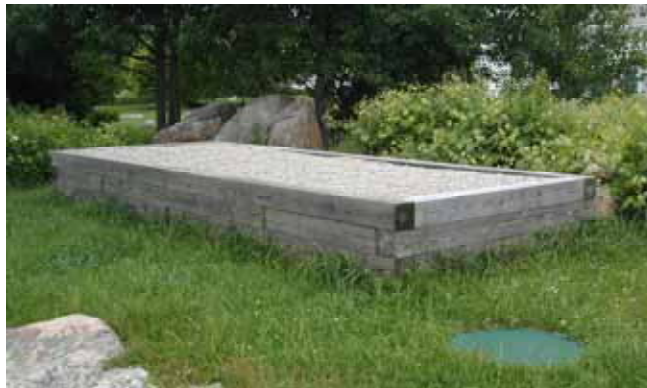
Figure 2-22 Raised Bottomless Sand Filter Following a Recirculating Media Filter (single-family home)
