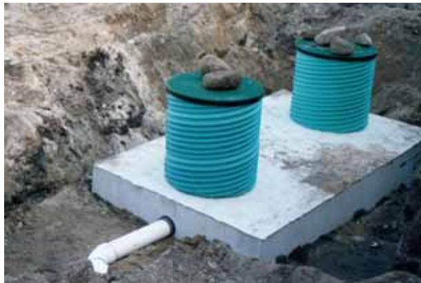
Figure 2-2 Concrete Tank with Access Risers Above Inspection Ports. When Backfilled, Riser Lids Will be at Ground Surface.
