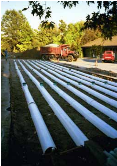
Figure 2-21 A Shallow Narrow Drainfield That Serves a Restaurant and Retail/Office Complex
