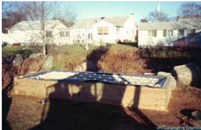
Figure 4-3 Bottomless Sand Filter Before the Final Cover of Peastone
