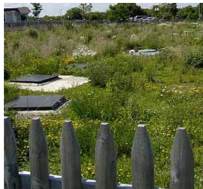
Figure 3-88 Lids Are the Only Parts of the System Visible from the Surface
