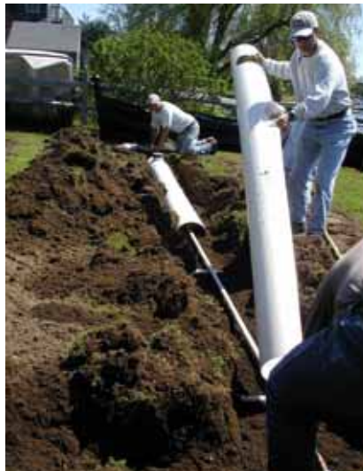
Figure 2-19 Installation of a Shallow Narrow Drainfield
