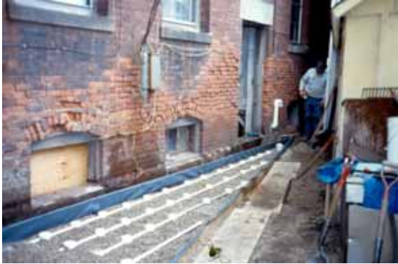
Figure 3-58 Bottomless Sand Filter Used as a Drainfield
