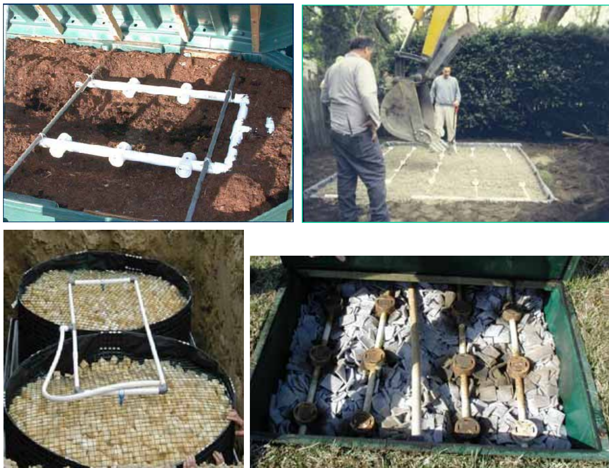
Figure 2-15 Examples of Media Filters: Peat Filter (top-left), Single-Pass Sand Filter (top-right), Foam Filter (bottom-left), and Textile Filter (bottom-right)
